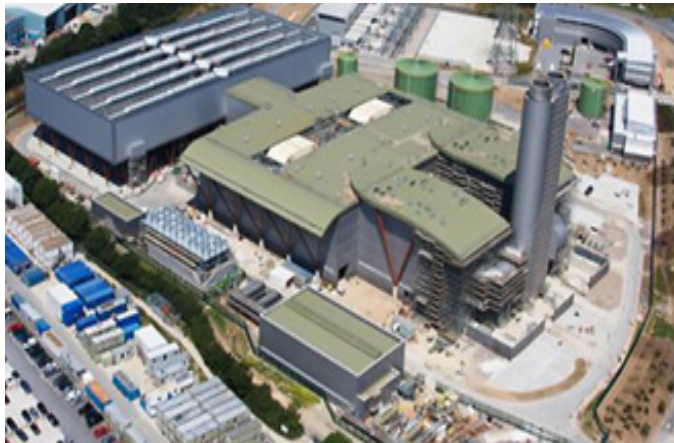
Administration and Support Buildings to support the £10m Langage Energy Park in the South West of England
